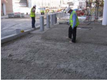
Shallow mounts before concrete
