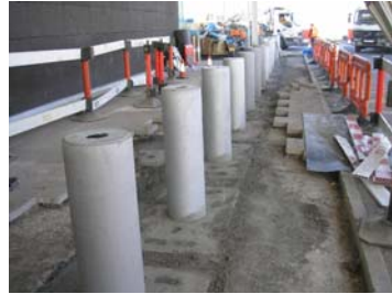
Shallow mounts after concrete
