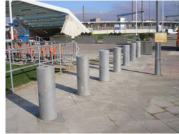
Shallow mounts after paving
